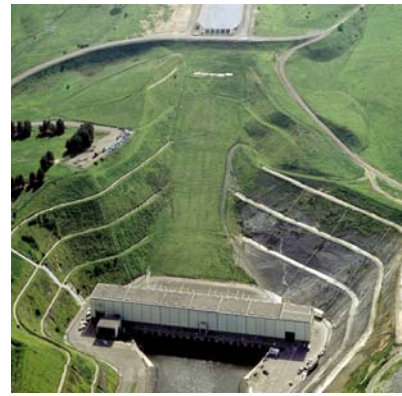
Banks Pumping Plant
