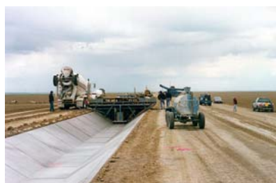
Canal Lining to Prevent Seepage Losses
